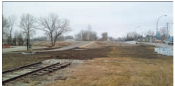
Figure 3 - Post office photo - Alberta, High River, main, levee on north side.
