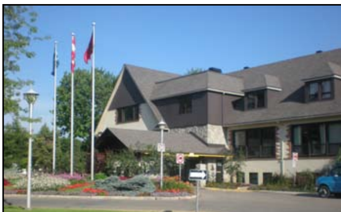
Sarto Desnoyers Community Centre
