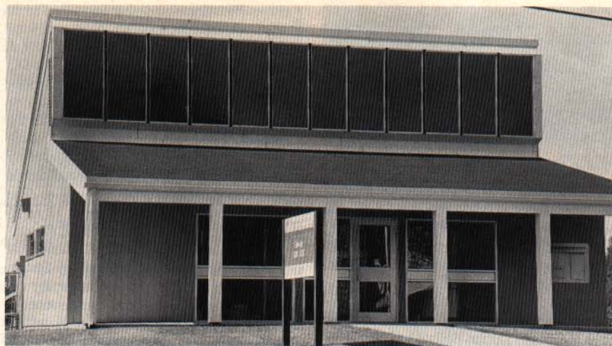
Greely ON post office showing 12 solar-heating panels
